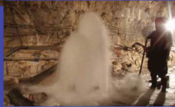
Water inflow from the bottom
