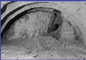
Typical appearance of a small karstic void partially filled with clay and silt; Dodoni tunnel, northwestern Greece, 2000.
